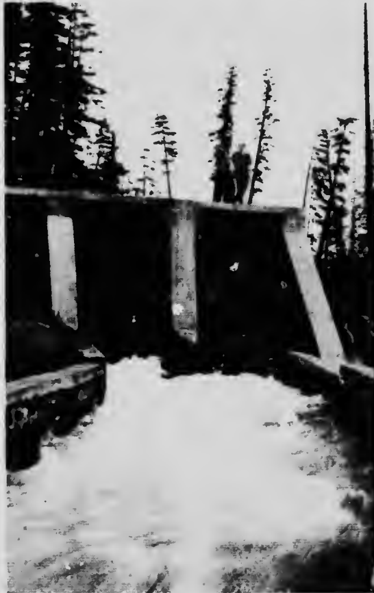
Canadian Collieries (Dunsmuir) Ltd. Flume Intake at Diversion Dam.
